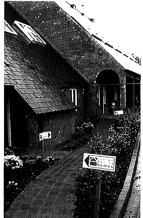
Partly completed apartments and show home at The Institute, Station Road.
